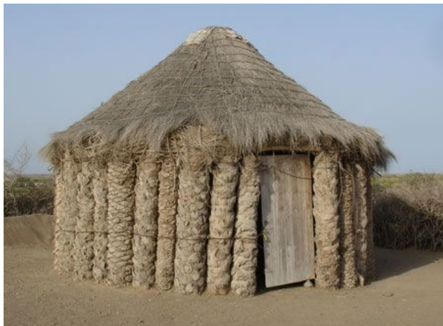
Fig. 13. Typical Tihama house, Palm trunk construction and thatched roof, Yemen, https://www.pinterest.com/artebitarealb/ (accessed September 28, 2023)
